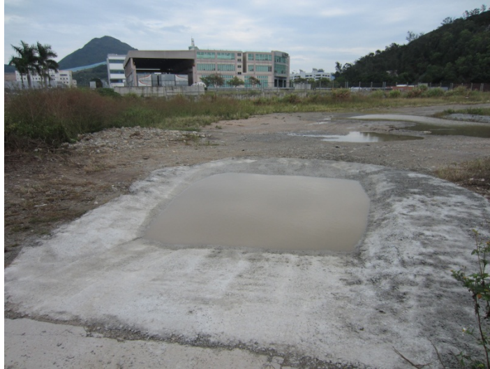
Photo 1 - A wheel-washing bay was available at the construction exit.
