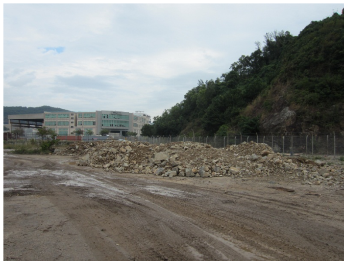
Photo 3 - Stockpiles of the excavated materials were observed to be exposed.
